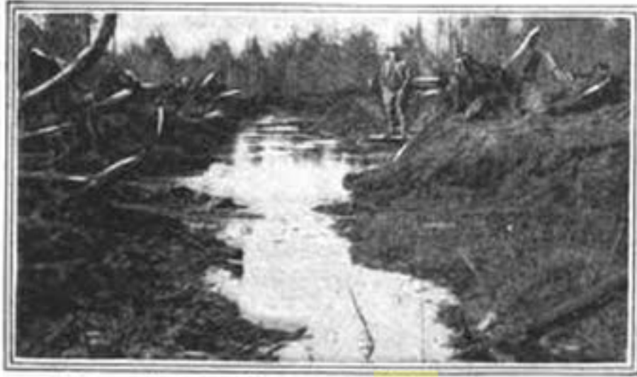
Figure 6—Image from Popular Science Monthly showing water filling the ditch on Kaufman’s farm immediately after blasting
