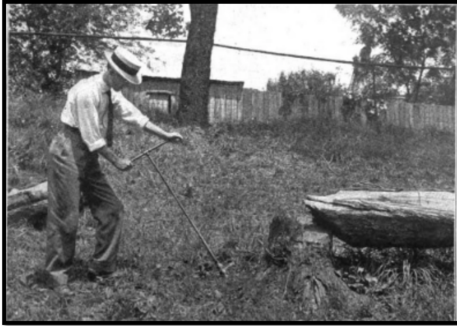
Figure 1: Kansas experiment station worker using an auger to create a hole under a stump to be removed with dynamite, circa 1911.
